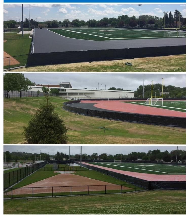
Images from top to bottom: Track base mat; track sealer; track sealer, different angle (May 2021)
