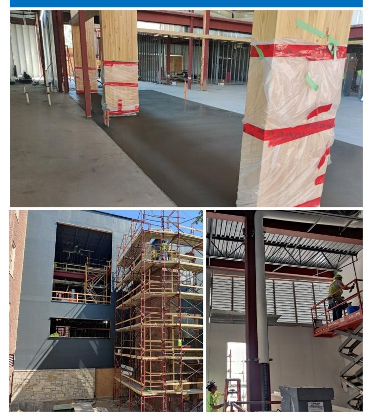
From top, then left to right: New concrete floor of administrative addition and Longhouse; stone base on the four-story connection (bottom left of photo) and link and brick work on the three-story addition (right side of photo); fresh air grille installed (top right of photo) and gypsum board being applied to second-floor mechanical space (May 2021)
